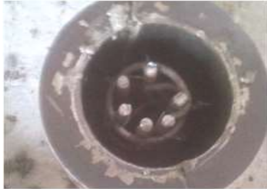
Figure 2 Cage placement in mould
